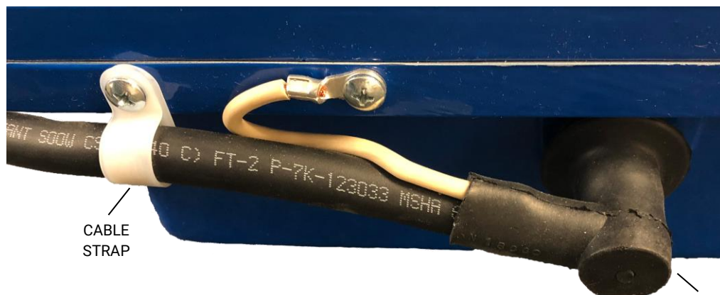
Grounding Cable Fully Installed
